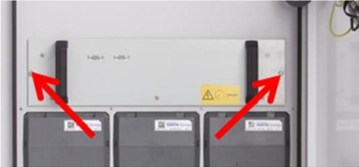
**Figure 27: Undoing screws on the battery inverter**
