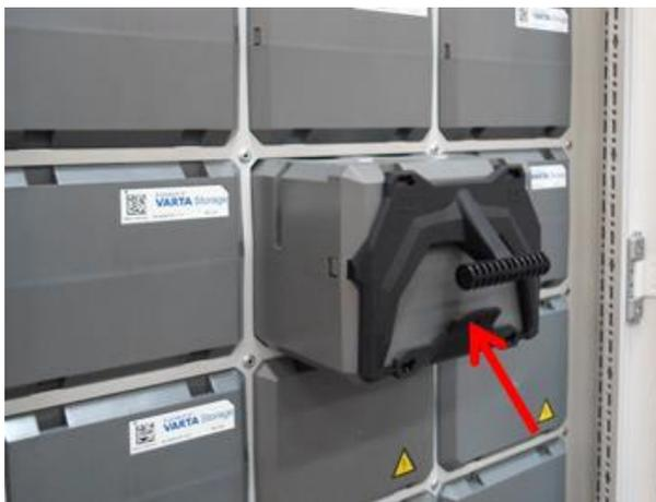
**Figure 34: Battery module with removal tool**
