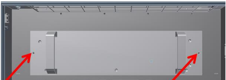
Figure 24: Undoing screws on the battery inverter
